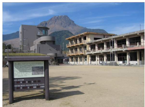
Fig. 5 Ohnokoba Elementary School building burned by pyroclastic flows on 15 September 1991. Back is the Heisei-Shinzan (lava dome formed in the 1991-1995 eruption). Courtesy of the Shimabara City.
