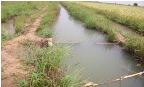
3. Tertiary canal (earthed).
