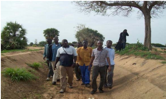
1. Canal panel (first area) overgrown with grass.
