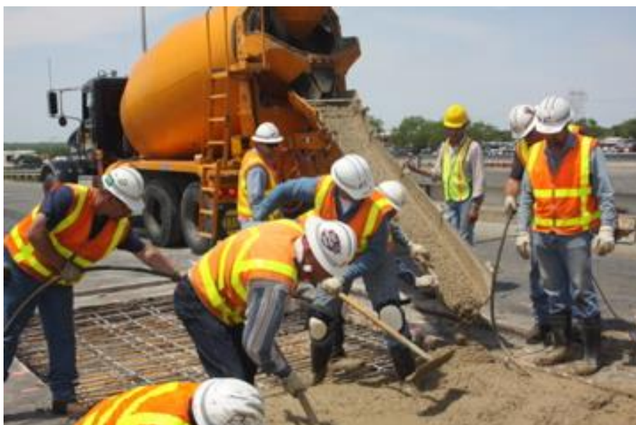
Fig. 5 Full depth repair, courtesy CeraTech, Inc., 2012.
