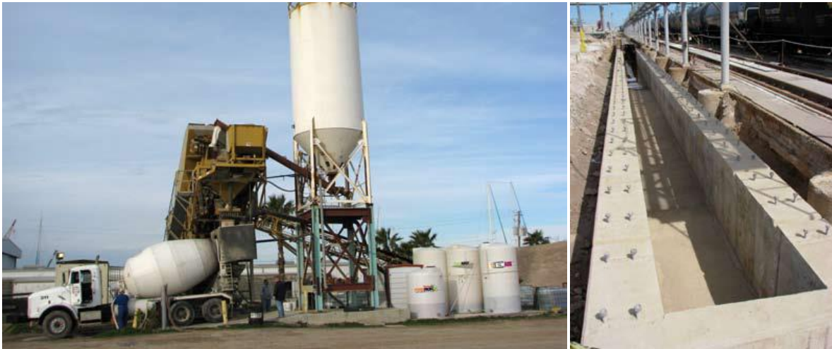
Fig. 4 Utilization of activated pozzolanic cement to prepare sulfur trenches, Galveston, TX. 2008, CeraTech, Inc.
